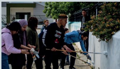
Local Ghardimaou Youth repainting the outside walls of the library
